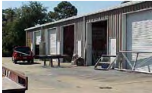
Storage Facility, Huntington Lane
